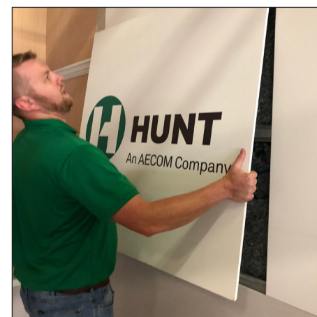
AECOM Hunt Project Manager of Preconstruction Aaron Sublette demonstrates how easy it is to remove a panel in order to access power and utilities behind the walls.
